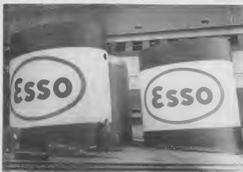
A PAINTER puts the finishing touches to prefabricated stacks for the "Esso Genova," "Esso Lima" and an upper bow assembly for the "Esso Suez."
